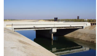
Bridge over the Faint-Kern Canal
