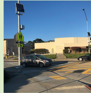
RECTANGULAR RAPID FLASHING BEACON
