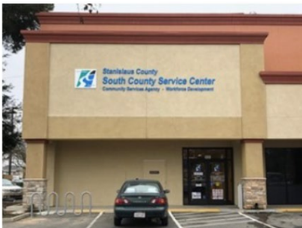
Turlock Office Pictured Above
