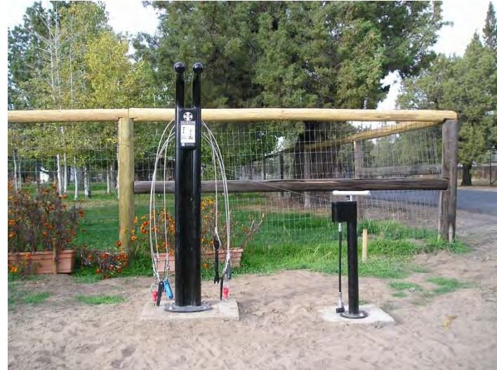
Example bicycle fix-it station on Twin Bridges State Scenic Bikeway, Oregon.
